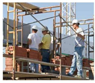
For smaller towers the equipment must be inspected after assembly, if an incident occurs that may affect the tower's stability, and at regular intervals. No-one expects a new inspection and report every time a mobile scaffold tower is moved around the site but if guard rails or other parts have to be removed then a pre-check should be undertaken by a trained contractor. The work at height act also requires contractors to record each inspection and use a visual tag system.
